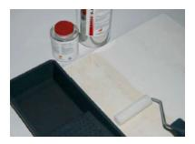
Note: Bonding of the panels is only possible after the prescribed drying time of minimum 12 hours.
